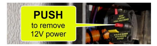
Note that when the red button is pressed, the yellow RESET lever flips down to the OFF position:
